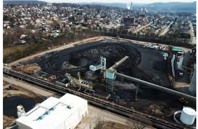
Former coal-fired Cheswick Generating Station in Allegheny County, Pennsylvania surrounded by residential neighborhoods. (Ted Auch | FracTracker Alliance, 2021)
